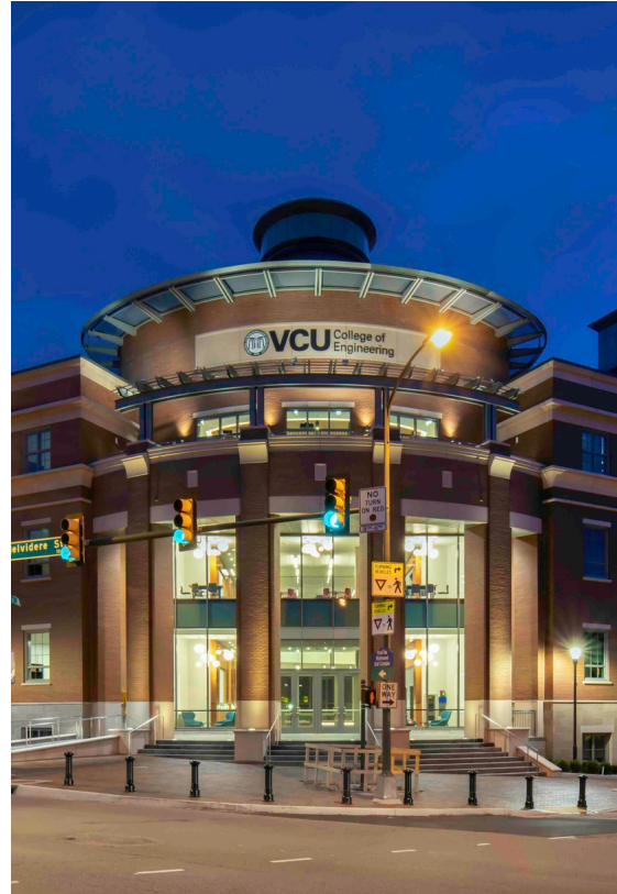
Engineering Research Building
