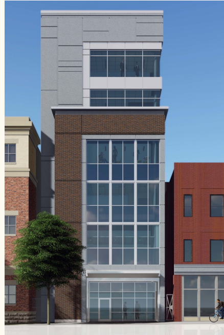
Technology Operations Center Under construction; estimated completion December 2023
