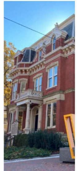
Founders Hall renovation
