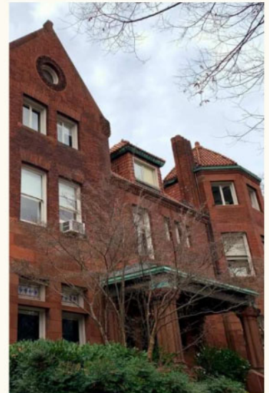
901 West Franklin Street renovation
